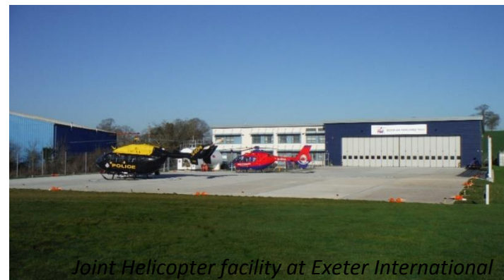
Joint Helicopter facility at Exeter International Airport
